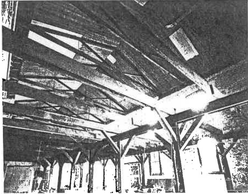
Removal of first floor section for Batavia Gallery.
